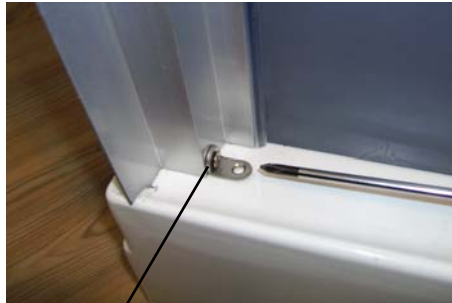
Použit šrouby 4,2x12 Svislé profily spojit s vaničkou use screws 4,2x12, link the vertical profiles with shower tray
