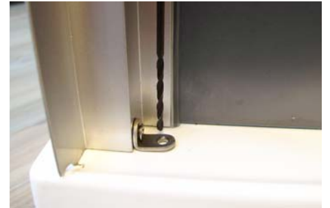
Vaničku vrtat vrtákem 3,2 mm drill the shower tray with 3,2mm drill
