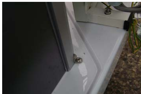
Použit šrouby 4,2x12 Svislé profily spojit s vaničkou use screws 4,2x12, link the vertical profiles with shower tray
