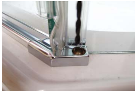
Vaničku vrtat vrtákem 3 mm drill the shower tray with 3mm drill
